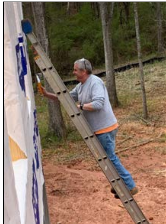
Shawn McGee installing housewrap.
